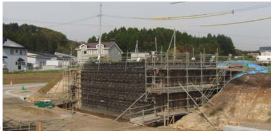
Fig. 33. The first full-scale GRS integral bridge, for the new bullet train line, at Kikonai, the south end of Hokkaido: a) overall dimensions (by the courtesy of Japan Railway Construction, Transport and Technology Agency); and b) a picture of the east side abutment, 14 th October 2011.
