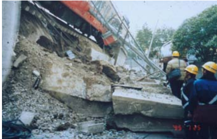
Fig. 10. Gravity type RW without a pile foundation at Ishiyagawa that collapsed during the 1995 Kobe Earthquake (Tatsuoka et al., 1997, 1998).
