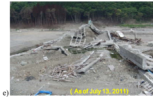
Fig. 19. Embankment-type coastal dikes; a) typical cross-section (Technical research group of coastal protection facility, 2004); and the concrete slab at the crest and the top concrete panel facing on the downstream slope lifted up and washed away followed by erosion of the backfill, caused by overflow of tsunami; b) Koshikiri, Sanriku-cho, Ohunato City; c) Tsugaruishi, Miyako-minami (note: the full-section of dike was lost at sections close to these sites); and d) & e) west of Bentenzaki, Aketo, Tanohata village, Shimo-hei gun, Iwate Prefecture.
