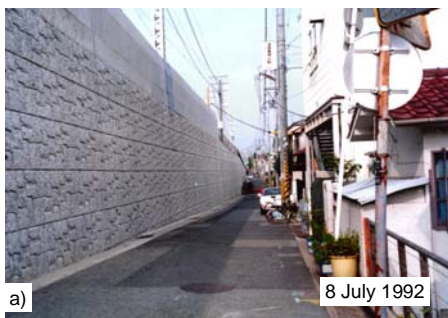
Fig. 10. Gravity type RW without a pile foundation at Ishiyagawa that collapsed during the 1995 Kobe Earthquake (Tatsuoka et al., 1997, 1998).
