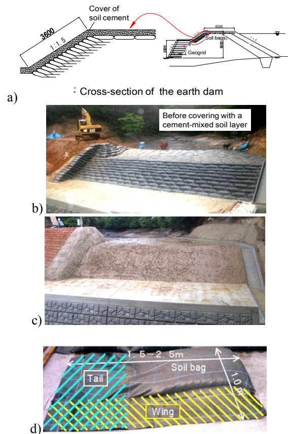
Fig. 18. Restoration of the earth-fill dam of Hirata Ike, Ishikawa Prefecture, that collapsed by the 2007 Noto-Hanto Earthquake (Mohri et al., 2009).
