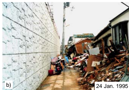
Fig. 11. GRS RW having a FHR facing at Tanata; a) immediately after construction; and b) one week after the 1995 Kobe Earthquake (Tatsuoka et al., 1997, 1998).
